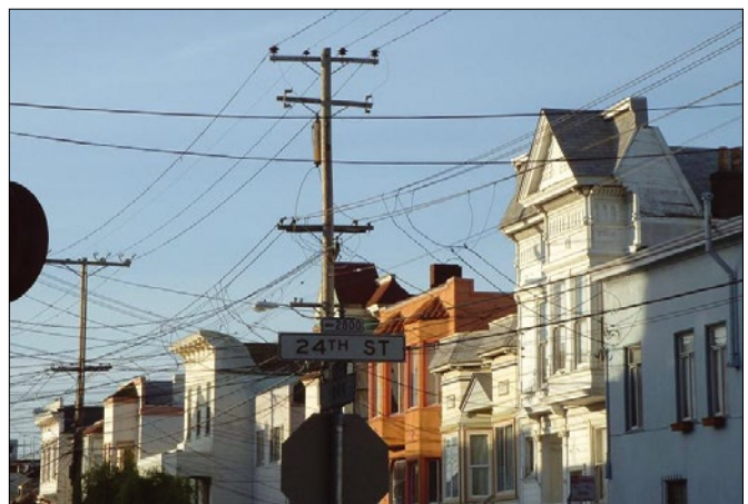
Figure 1: San Francisco: Supplying power through a bird's-nest of cables can lead to failure.
