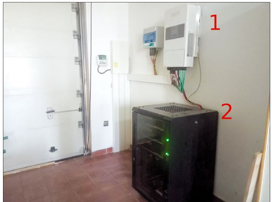
Figure 2: A Turbo Energy hybrid inverter (1) paired with a battery bank in a rack (2). The photovoltaic panels charge the batteries with excess production, so the owner can use battery power after the sun sets.
