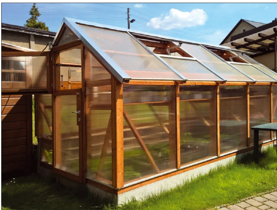
Figure 1: The automatic greenhouse control system regulates when the skylights open and close.
