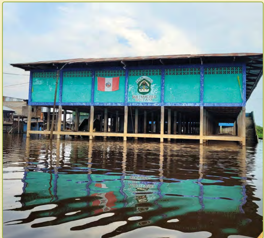
■ The San Francisco Rio Itaya School is built two stories up on stilts because flooding is an annual event in the lower section of Belén, Peru
